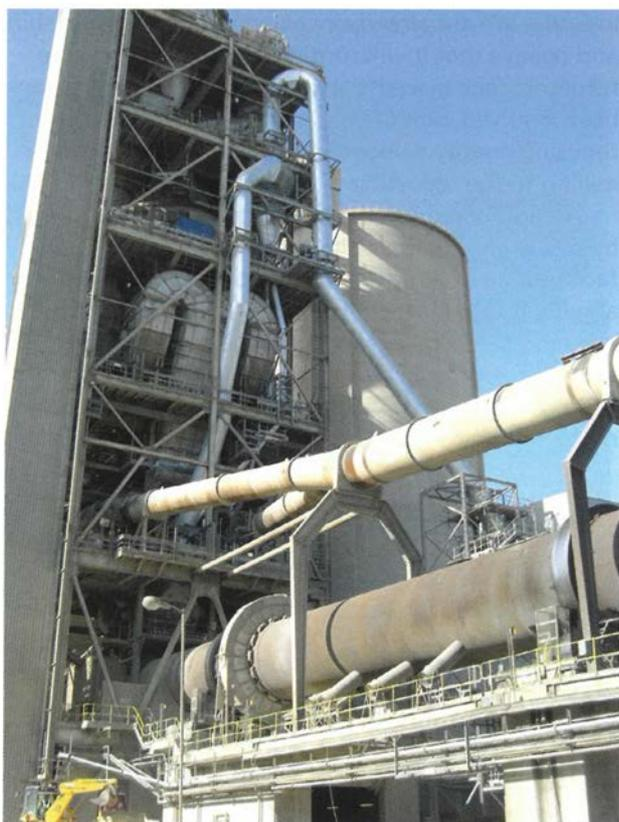
Kiln bypass at Ketton cement plant.
