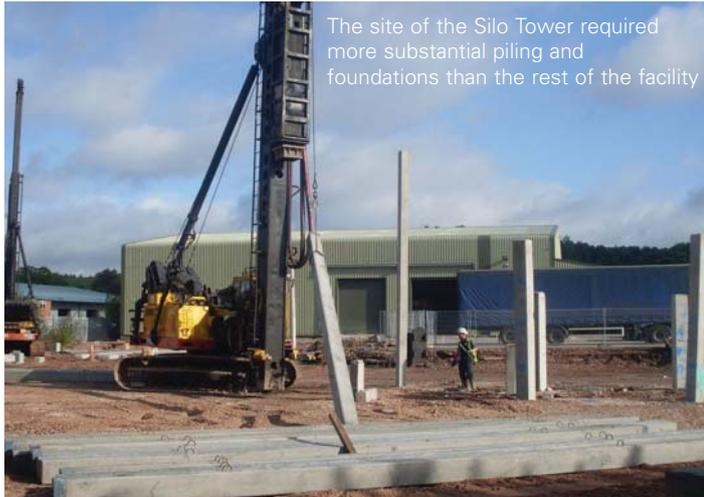
The site of the Silo Tower required more substantial piling and foundations than the rest of the facility
