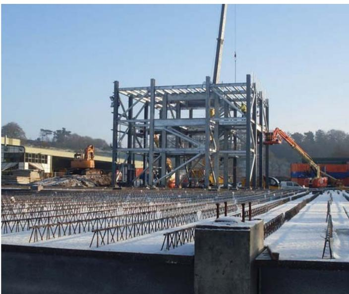
During the early stages of the Silo Tower construction various key pieces of equipment needed to be installed as progress was made – screw conveyors, weigh hoppers and the mixer – in order to allow the structural construction to proceed in an effective manner.
