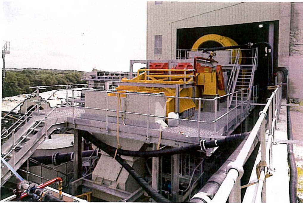
After washing the material is separated into gravel and finer fractions of clay, sand and mica
